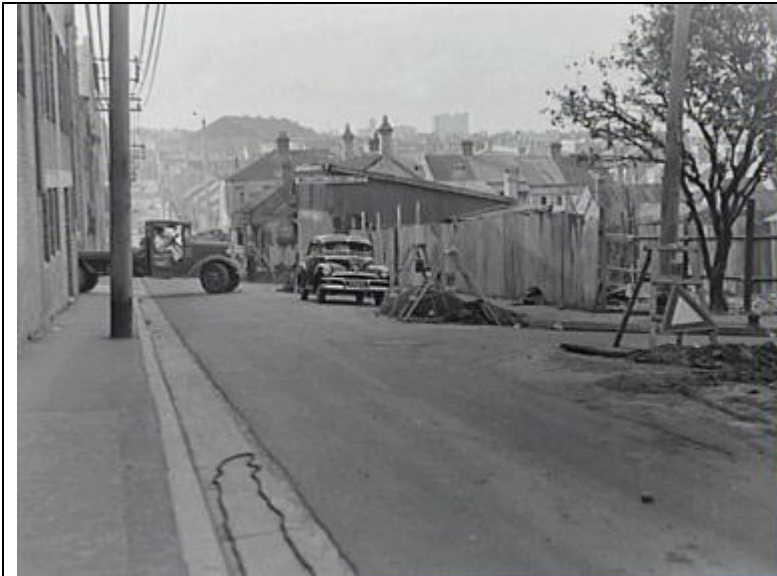
File: 010\010498 Title: Angel Street Newtown – looking north to the Erskineville Road end. Date: 6 August 1956 Citation: NSCA CRS48/498
